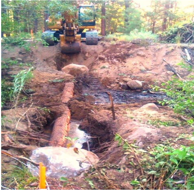
Restoration of Third Creek, Incline Village, NV
